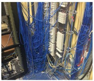
**FIGURE 10.12** Tracing Ethernet cabling 2.
